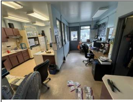
Samples: LFL01-B Description: FT1 - Floor Tile 12x12 Note: Floor tile w/ adhesive
