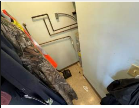
Samples: LFL01-A Description: FT1 - Floor Tile 12x12 Note: Floor tile w/ adhesive
