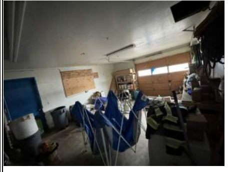
Samples: LF01-A Description: Mortar / Joint Compound Note: Concrete poured foundation
