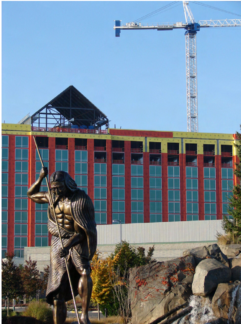
The hotel expansion at the Tulalip Resort Casino
