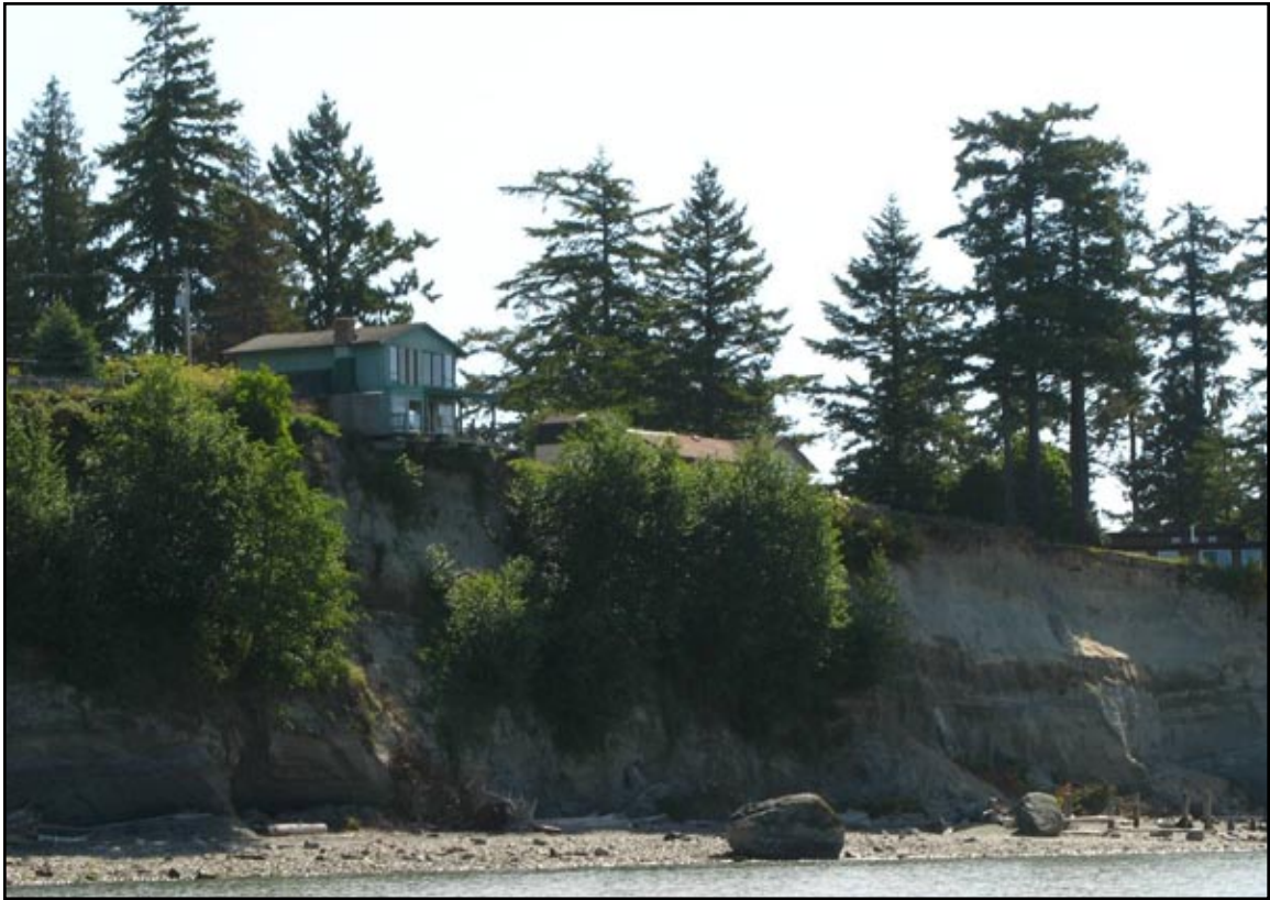
Figure 13: Vulnerable Homes on Hermosa Point
