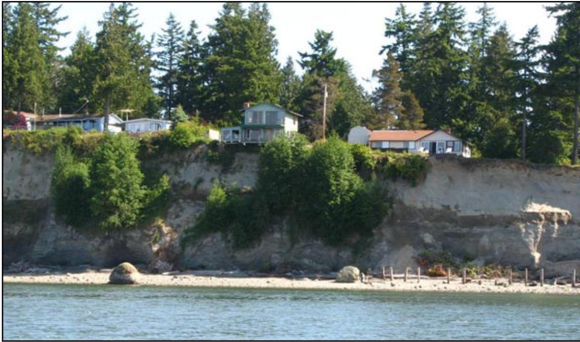
Figure 11: Vulnerable Homes on Hermosa Point
