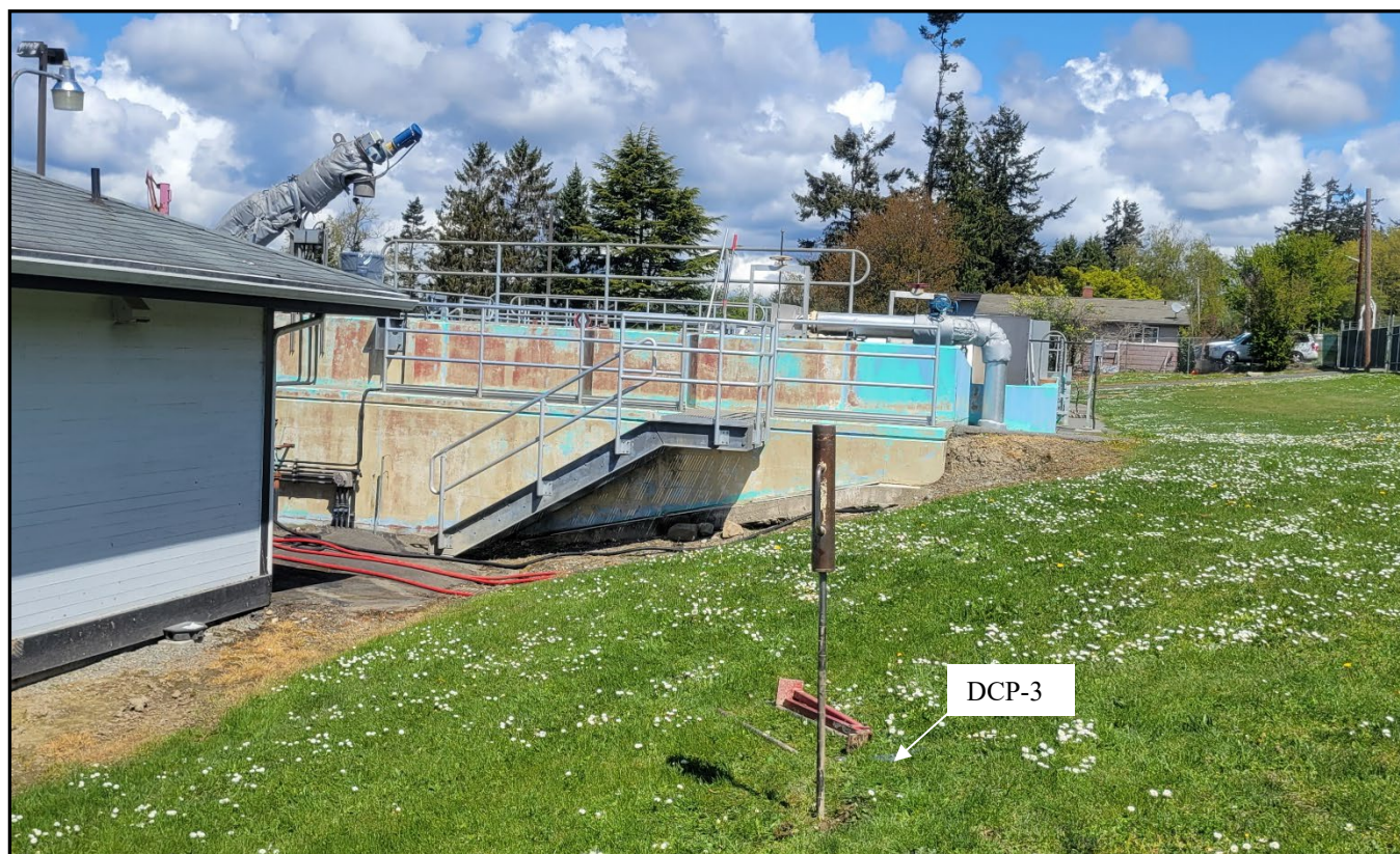
Photo C: Looking north DCP-3 in progress.
