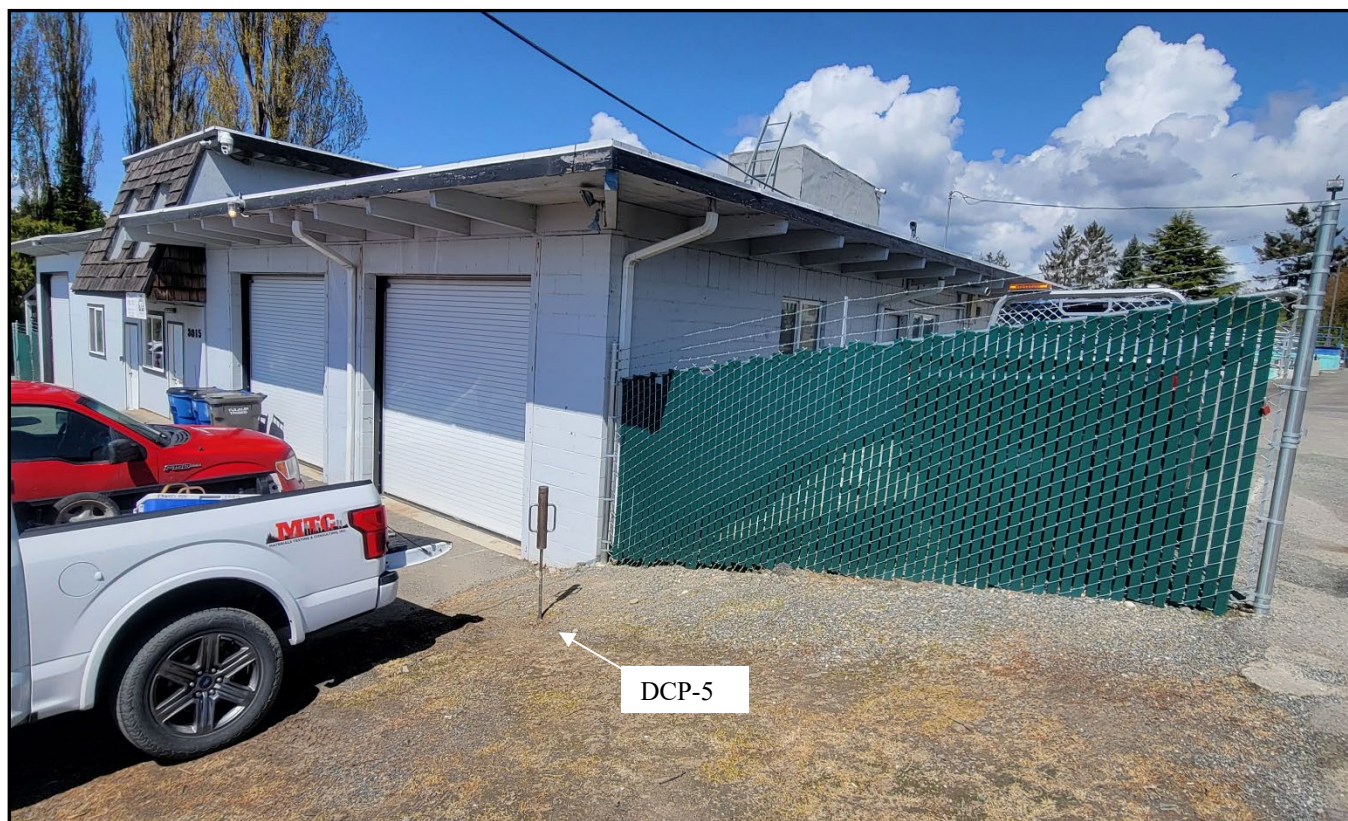
Photo D: Looking north at the southeast corner of the building. DCP-5 in progress.
