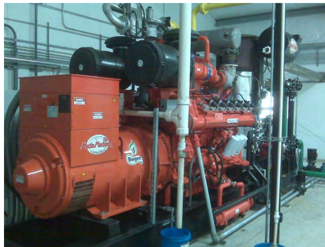
Figure 10. 450 KW generator run on methane to produce electricity.
